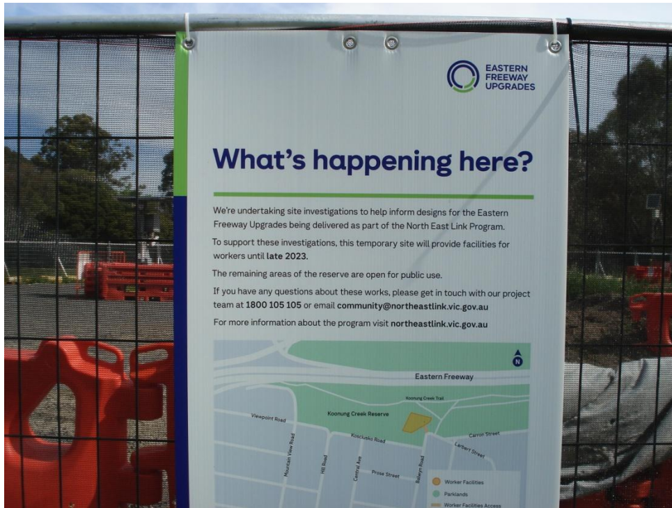
Photograph 15: Sign displayed on site compound fence near Kosciusko Road, Balwyn North. Breathtaking hypocrisy shown here - “Site Investigations for Freeway Upgrades”. No mention of tree or wetlands loss or destruction of parkland!”
