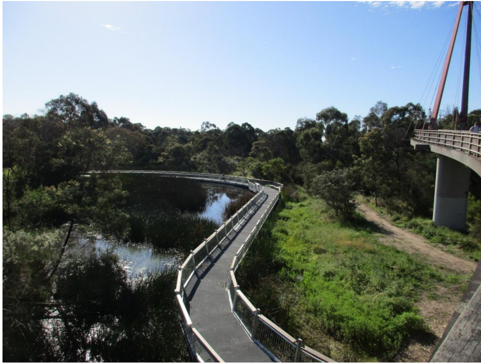
Photograph 7: View of Koonung Creek wetlands, Mont Albert North with pedestrian bridge over Eastern Freeway on the right
