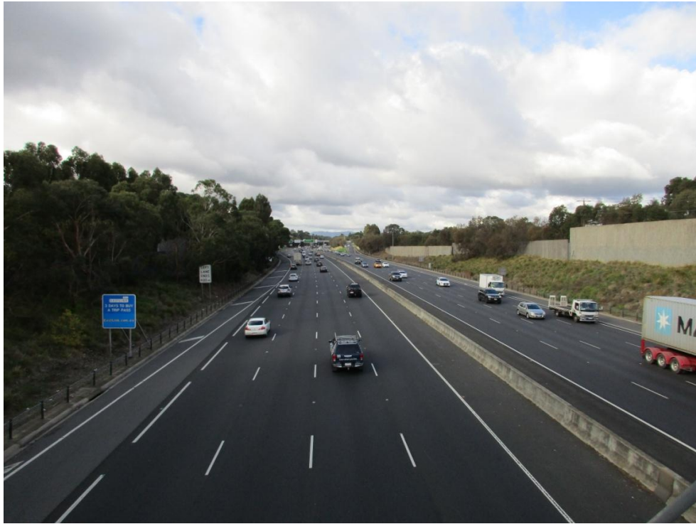
Photograph 17: Eastern Freeway traffic sewer at midday looking east towards Blackburn Road. Note reasonably well treed and landscaped road side, all to be presumably lost in a road widening concrete canyon similar to most other Melbourne freeways.
