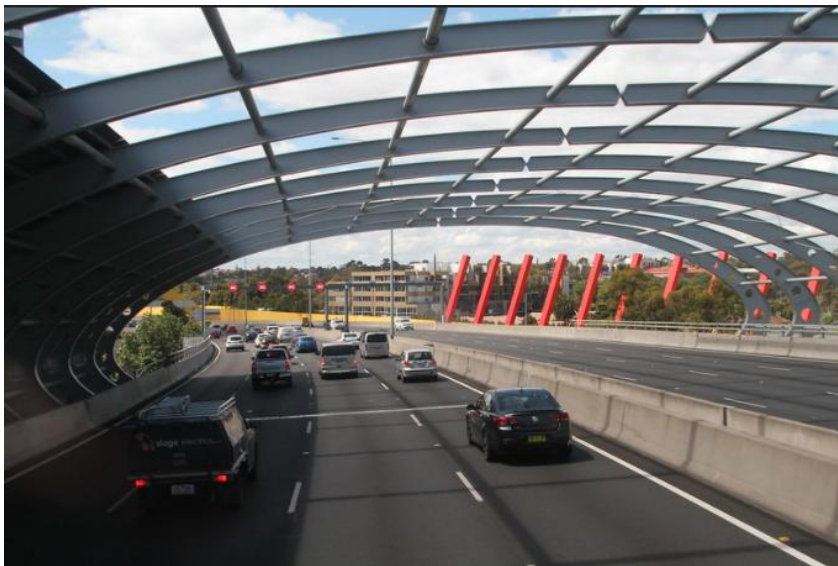
Figure 5. Bolte Bridge sound tube
